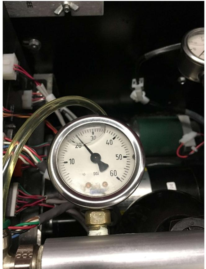
3.) The GUI screen Oil Pressure reading must match with the gauge reading. If the Oil Pressure GUI reading is below the gauge reading, or if the GUI Oil Pressure reading reads anything between -1 to -8 when the gauge reads 0 please replace the pressure sensor.
